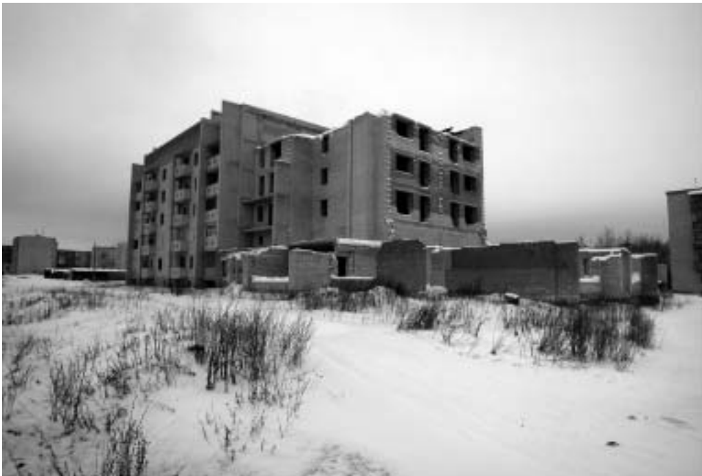
Foto 4: Yuzha – unvollendeter Wohnblock / Unfinished Tower block. © Philipp Oswalt.
